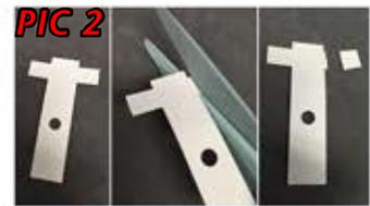
**Step 3.** Locate the t-shaped gasket that came packaged with your outlet. Cut one of the sides off.
